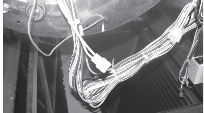
Figure 12: Install Two Pin Jumper Plug
